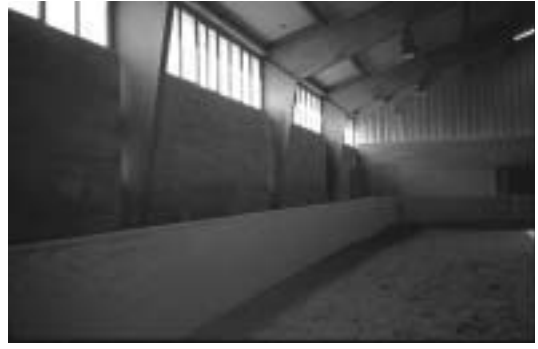
Figure 3.3. Rigid frame clear-span construction is more common in wide indoor arenas than in stables.
