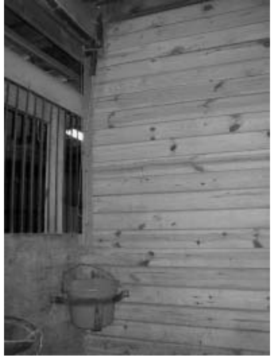
Figure 2.14. Labor-saving features and efficient routines are important because of the high labor demands of horse housing. This stall features a labor-saving overhead water line that supplies the bucket with water after a valve is manually activated.
