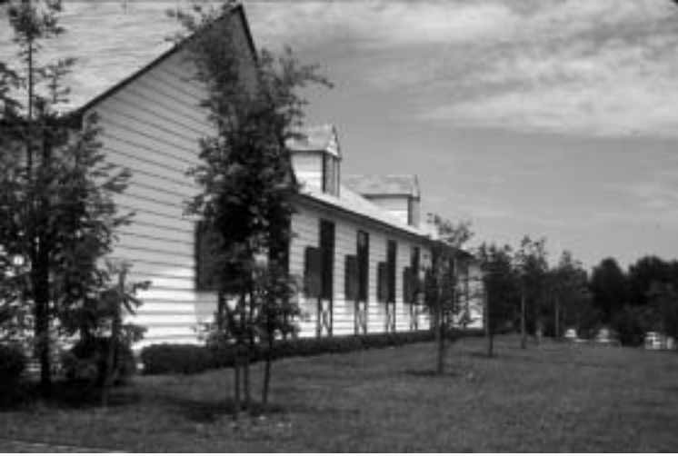
Figure 2.1. Housing the horse in a stable offers many conveniences as long as management of interior environment and horse exercise is sufficient.
