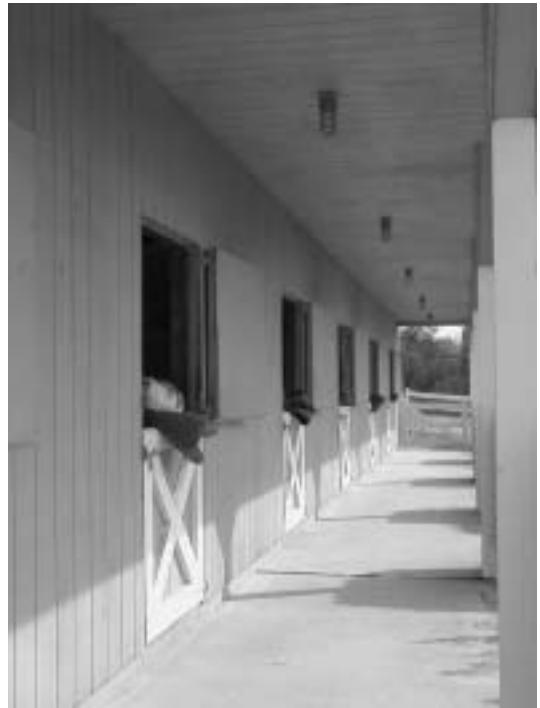
Figure 2.4. Single-row stall options are typically open to outside work aisle and are a good option in mild climates.
