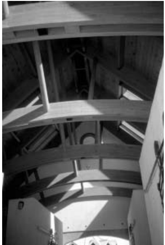
Figure 3.4. Wooden arches of glu-lam construction offer an attractive framing in simple rigid frame style or the more complex formation shown here.
