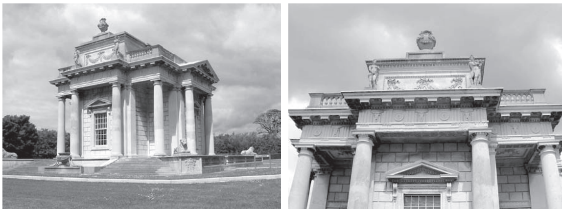
Figure 1.2 The Casino at Marino, Dublin, by Sir William Chambers, 1764. The urn is a chimney.
