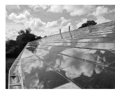
For the Smithsonian Tropical Research Institute Field Station Laboratory at Bocas del Toro in Panama, the design team first challenged criteria, divided functions to minimize loads, and created this large photovoltaic panel canopy that provides added shading and diffusion of light entering the occupied spaces below, as well as generating the majority of energy required for this laboratory facility. *Image courtesy of Kiss + Cathcart, Architects.*
